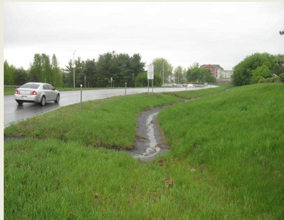
I-89 Exit 14 - enhancement needed to address paved swale
