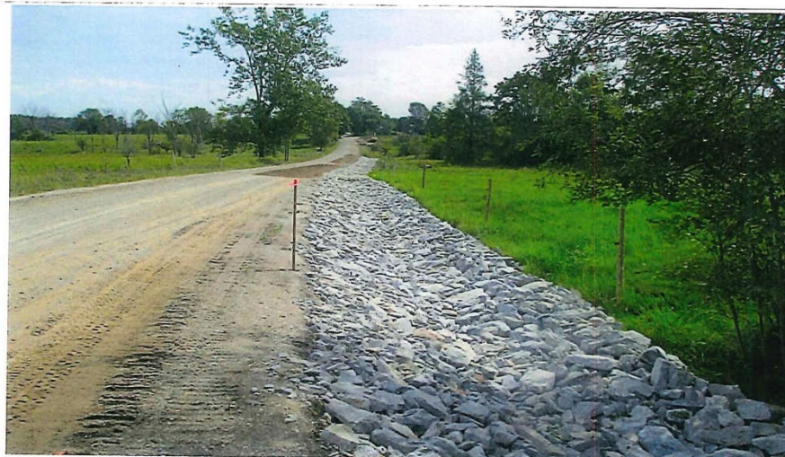
Fairfield, VT After
